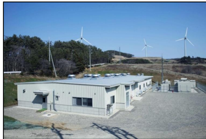
Electricity storage facilities for wind power generation (Ichiura Wind Power Generation Plant)
